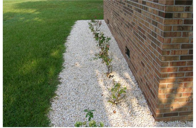
**Figure 8. Use inorganic mulch, such as decorative gravel, around buildings whenever possible to eliminate potential harborage areas for pests.**
