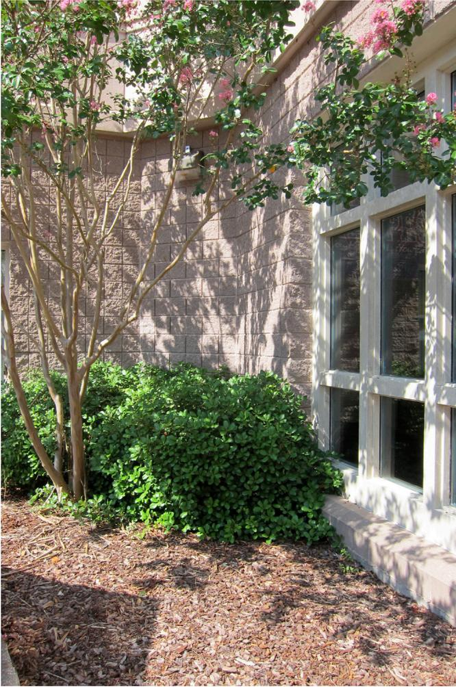
**Figure 7. Branches and limbs that touch buildings should be trimmed back so that ants and other insects cannot use them to access buildings.**
